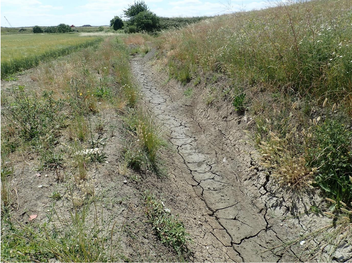
Figure 20: Newly dug section of Ditch D10.
